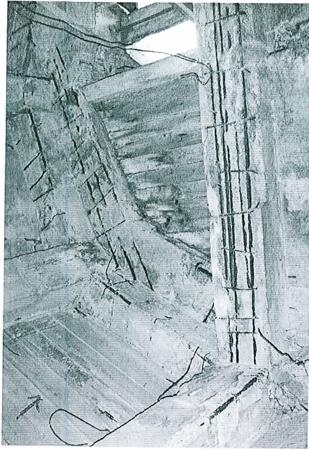
Turn central interior (in pod)
