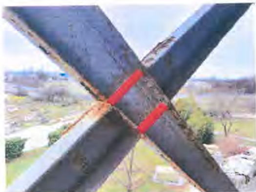
Fig. 1: Continuitate tălpi profile UNP140
