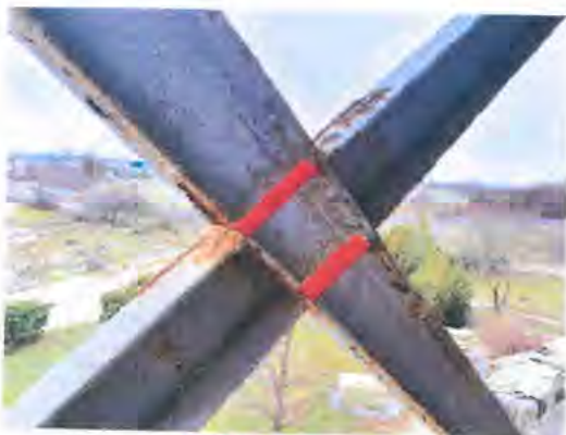
Fig. 1: Continuitate tălpi profile UNP140
